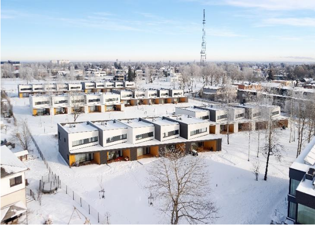
Terraced houses at Vaarika 1a, 1b and Tammepärja 17, 19 (contractor: Embach Ehitus OÜ, photo: Karl Kasepõld)
