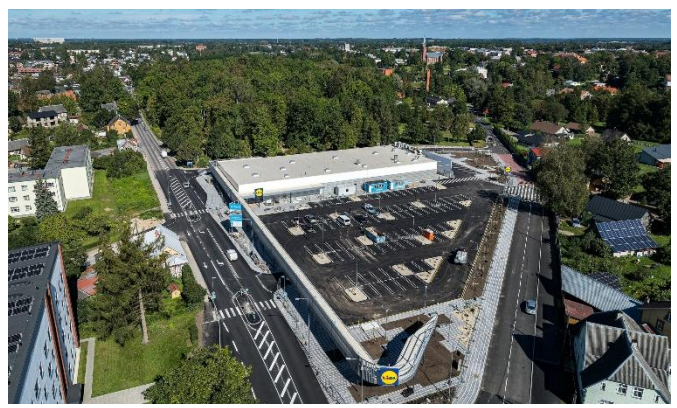
Lidl store in Viljandi (contractor: Embach Ehitus OÜ, photo: Kristjan Lust)
