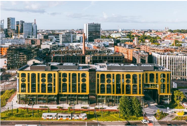
Golden Gate office building (contractor: Nordecon AS, photo: Kaupo Kalda)
