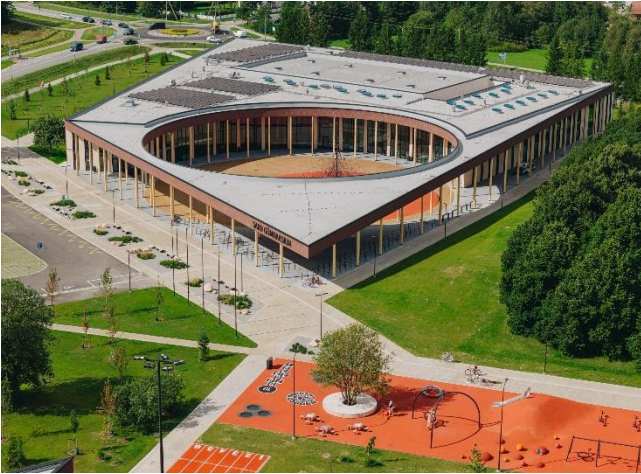
School building and sports complex of Saku Upper Secondary School (contractor: Nordecon AS, photo: Tõnu Tunnel)
